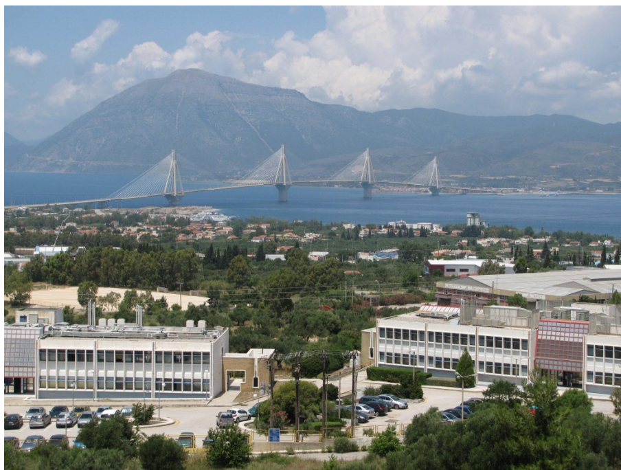
Figure 1: Outskirts of Patras near the Science Park, with the Rio–Antirrio bridge to mainland Greece in the background
